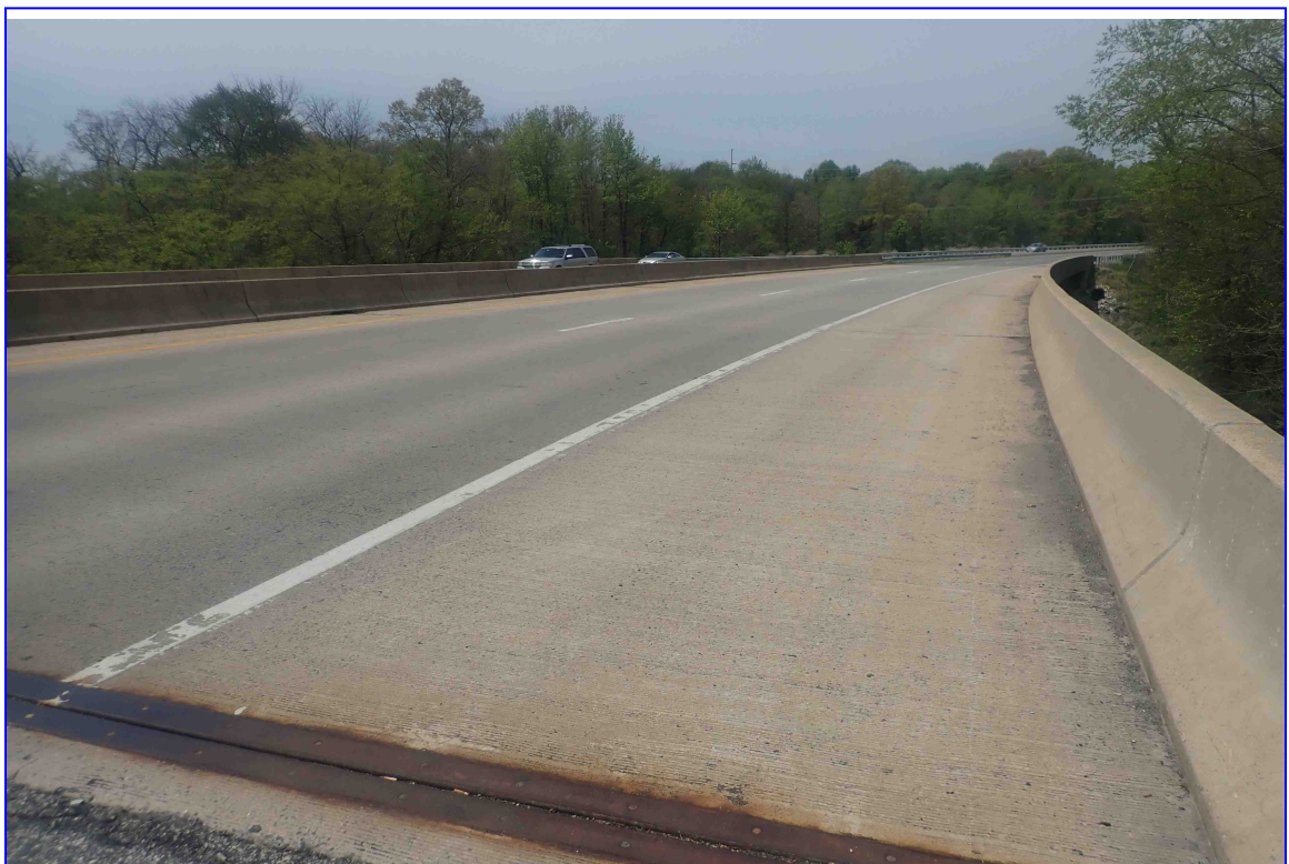
6. CONCRETE DECK WEARING SURFACE LOOKING WEST
