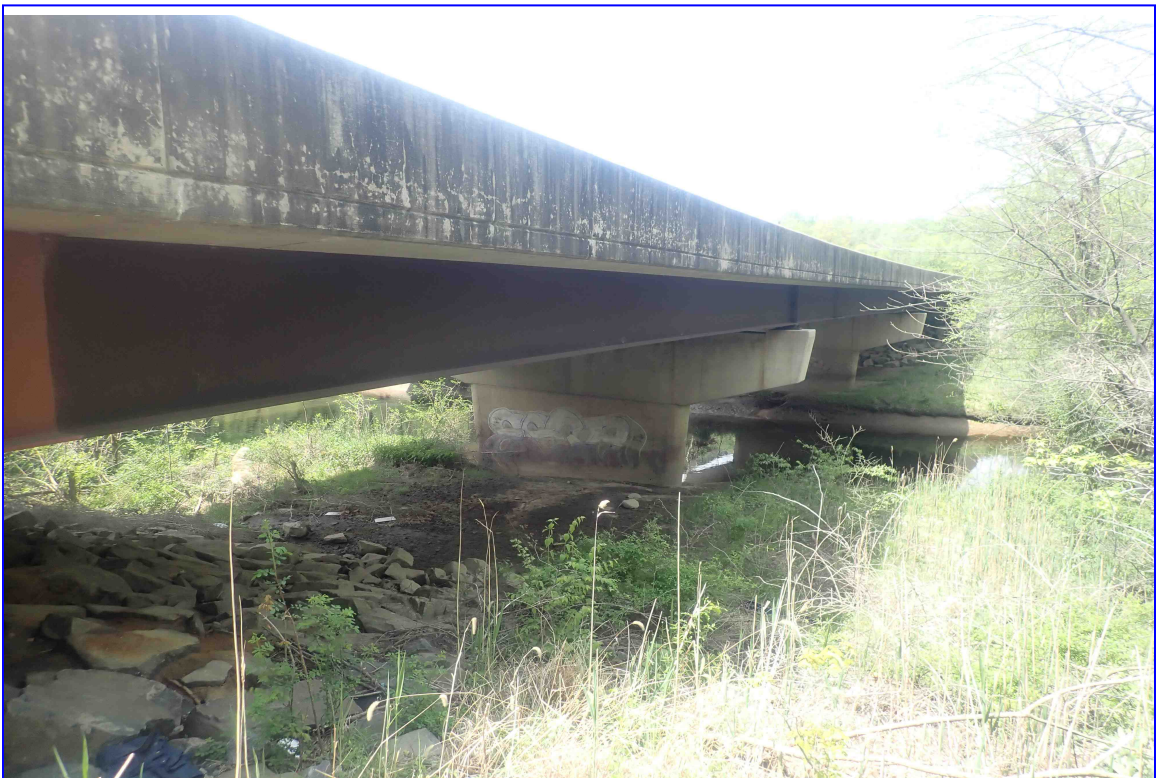
2. NORTH ELEVATION LOOKING SOUTHWEST
