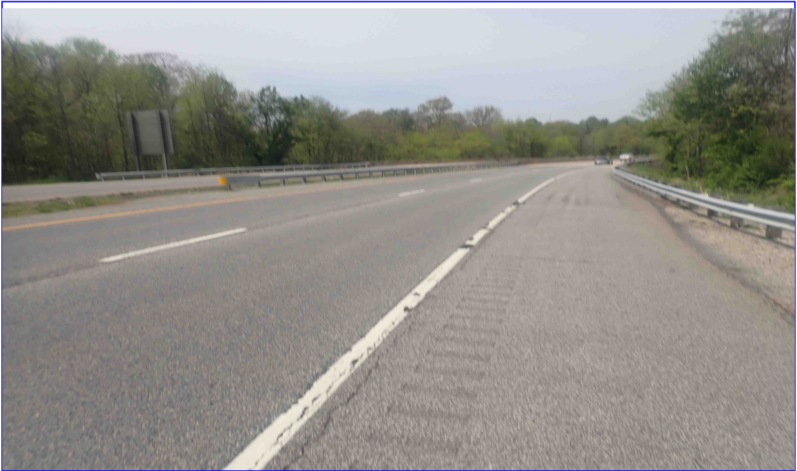
1. EAST APPROACH ROADWAY LOOKING WEST
