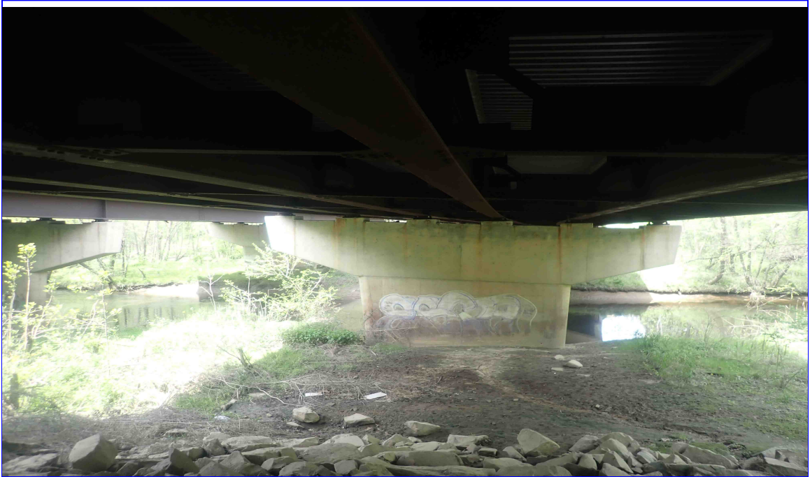
3. GENERAL VIEW OF SPAN 3, PIER 2 LOOKING WEST
